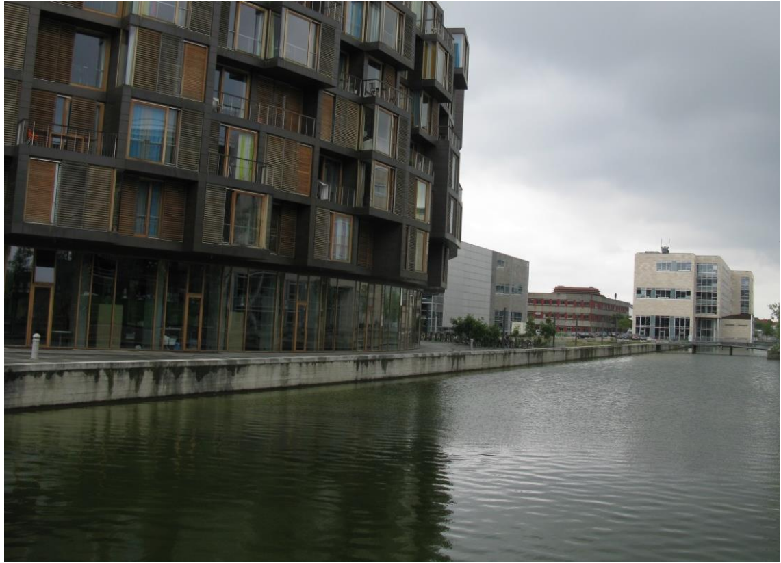
Figure 16. Open channel for storm water collection in Ørestad, Copenhagen.
